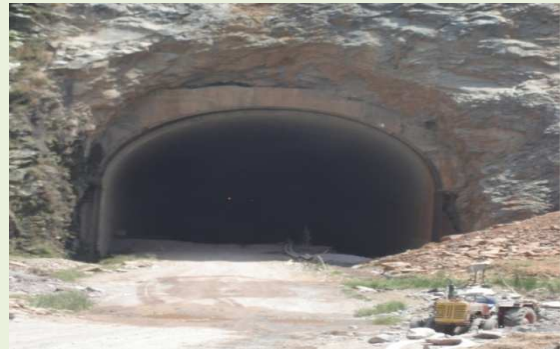
Tunnel work at Gandikota Reservoir under progress
