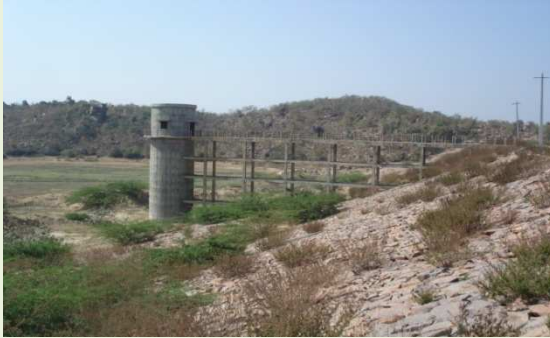
SS tank of Nyalkal scheme without water and without pumps
