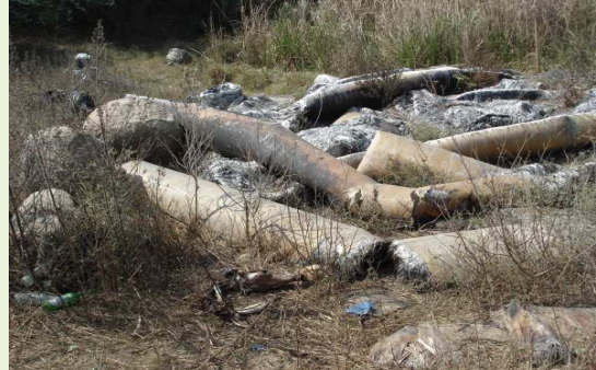
Burnt GRP pipes at the site relating to Part-IB works
